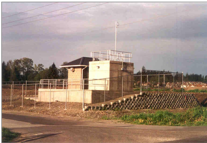
Morgan Creek Drainage Pump Station
