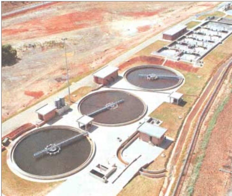
J.P. Marais Regional Sewerage Purification Work
