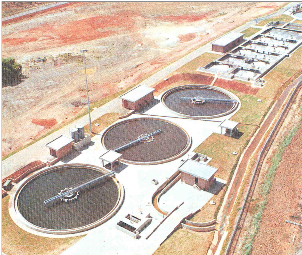
J.P. Marais Regional Sewerage Purification Work
