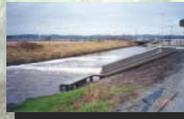
Photo No. 5 - Access Platform Over Flood Box Outlet.
