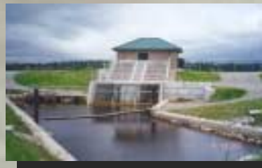
Photo No. 2 - View to the West. Showing Pump Station Inlet.
