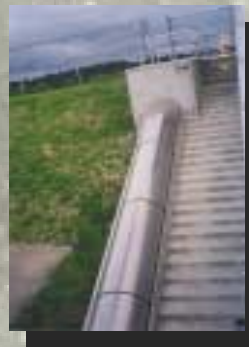
Photo No. 6 - Fish Ladder Chute Down to Forebay, with Aluminum Cover.
