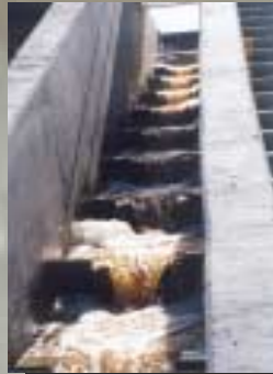
Photo No. 7 - Fish Ladder Rising Pools, Water Supply Flowing and Cascading Down in the Pools.
